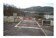
Moulinearn level crossing is protected by miniature red/green lights and audible warning equipment. An additional set of red/green lights has been provided on each side of the crossing, and there are restrictions on the use of the low-level barrier raise controls.
